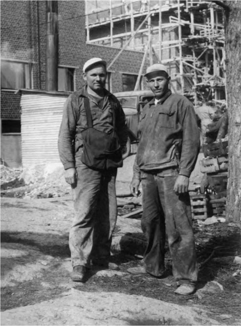
FIG 3.3 Antti (left) building the new paper mill in Sunila, Kotka
